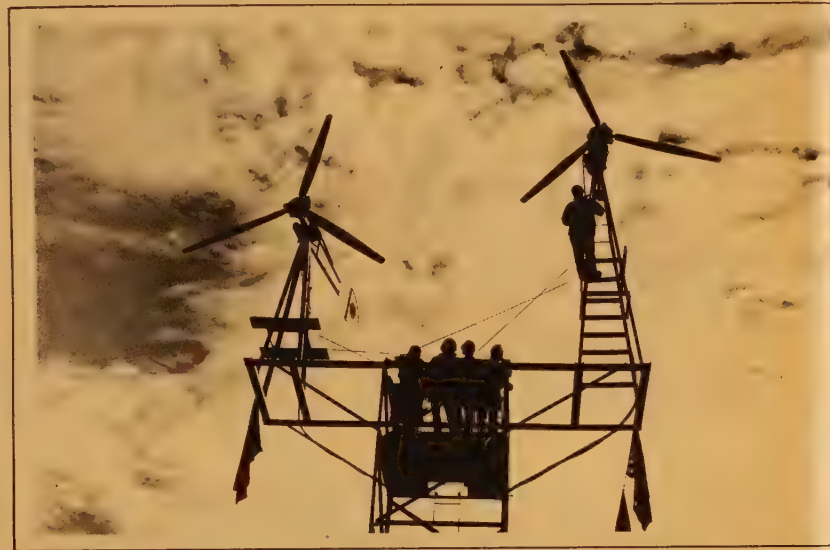
Twin Jacobs wind-electric plants at Integrated Living Systems, Albuquerque, New Mexico.
